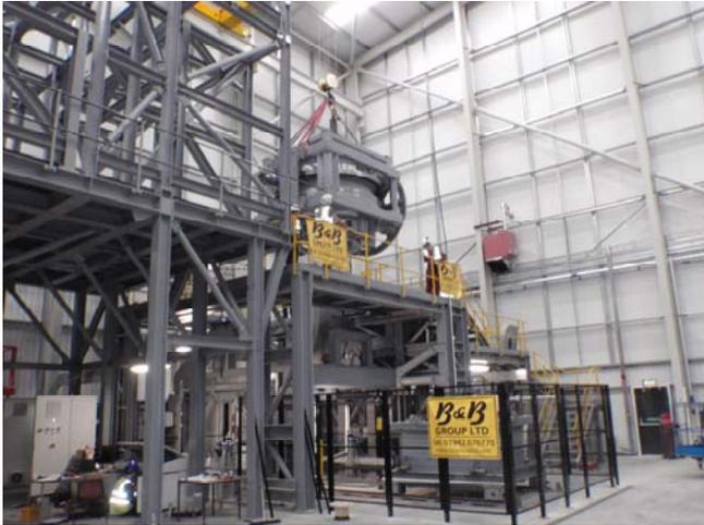
Installation of one of the Test Rigs undertaken to date, which has involved B&B undertaking the Principal Contractor's role, the management, design and build of various disciplines, including the piling and foundation works, the structural frame, the mechanical components, the EC&I works including the software management system, in accordance with nuclear specification standards as required by our client.
